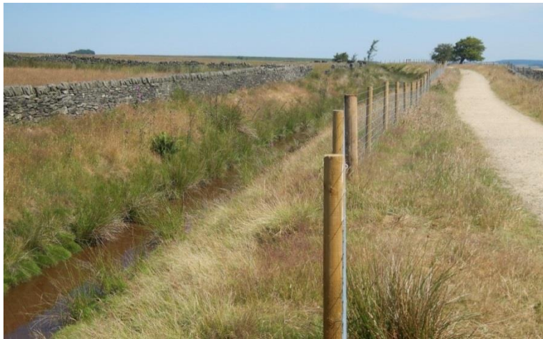
Figure 5. Fencing at Redmires Conduit
