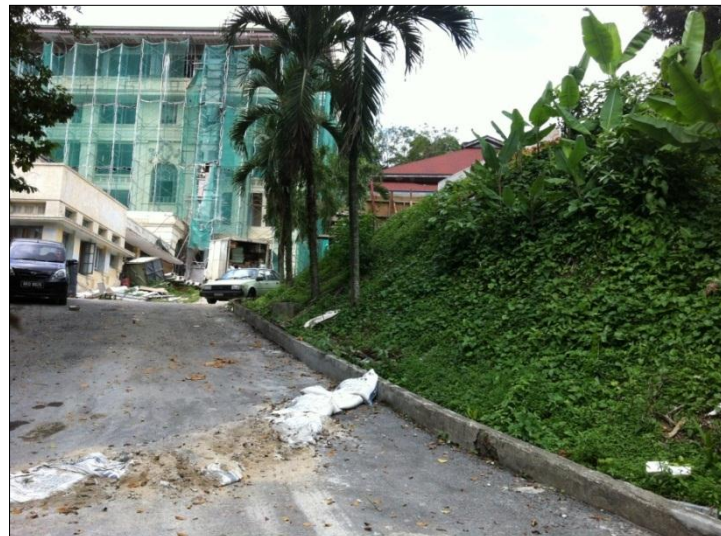
Figure 8: Hotel Majestic Kuala Lumpur during refurbishment works (Source: Author)
