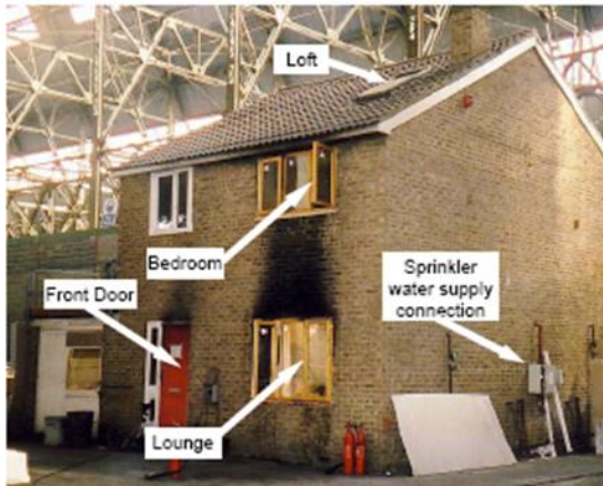
Figure 2 - Photograph of test house (BRE 2004)
