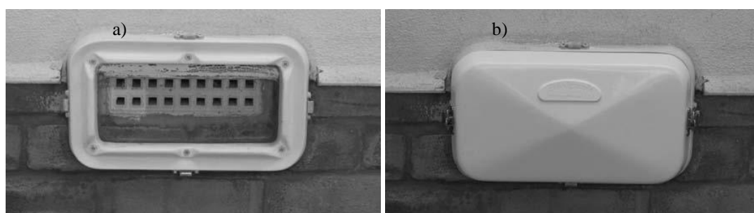
Figure 3: Images of an air brick with a surrounding fitting in place under normal operating circumstances (a). When a flood warning is in place this can then be sealed with the cover (b). Source: (Garvin, 2005 p. 61)
