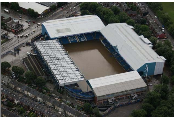
Figure 1. Flooding at Hillsborough Stadium (Image from Peter Smith, 2010)
